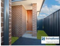
Tahmoor 14A Macquarie Place
