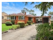
Tahmoor 9 King St
